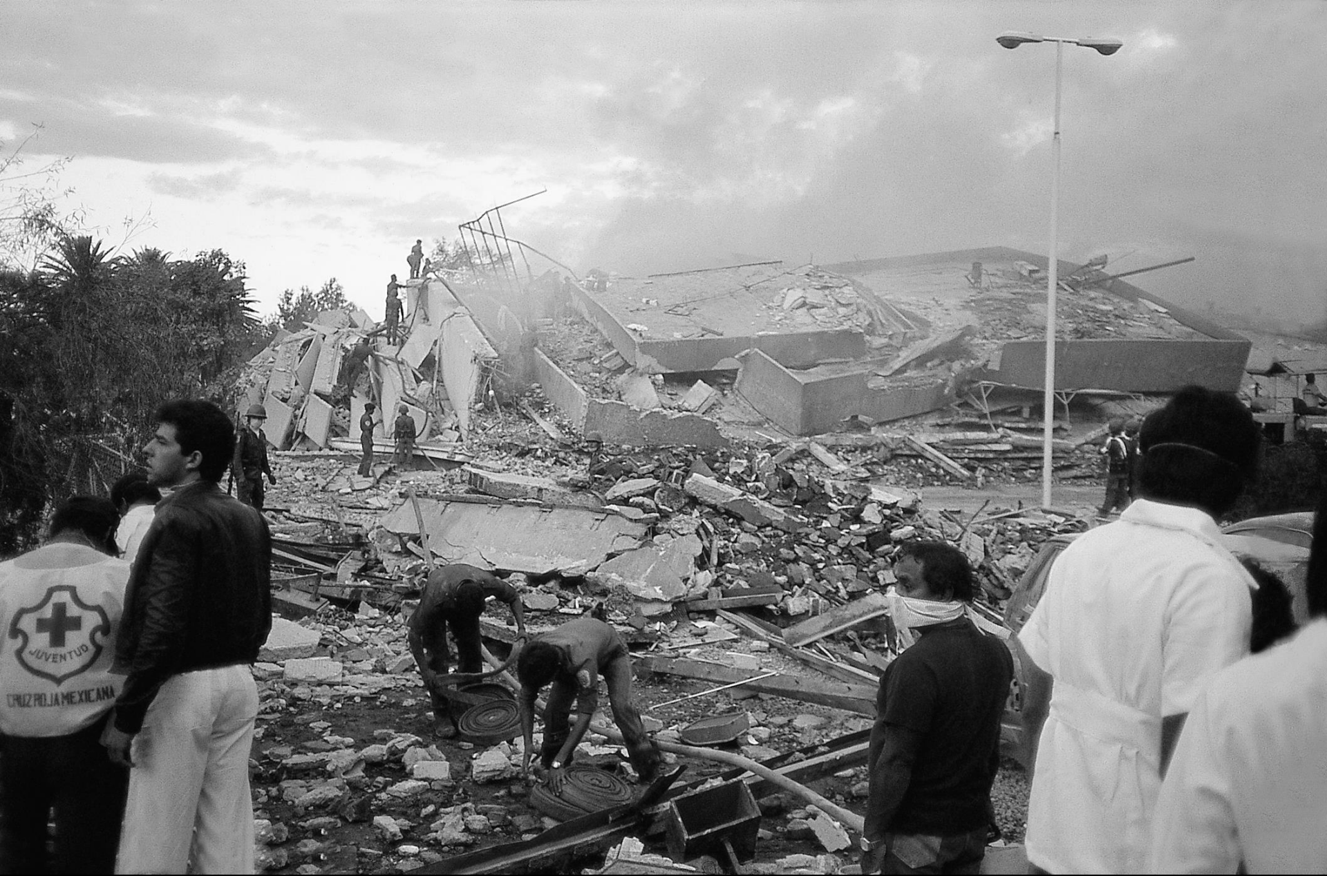
Hospital de Ginec Obstetricia del Hospital General de México
