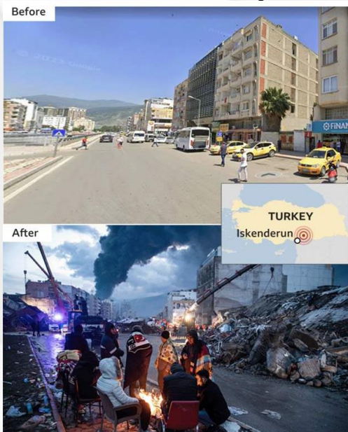
Edificio colapsado en Iskenderun Collapsed building in Iskenderun Fuente/Source: BBC Images
