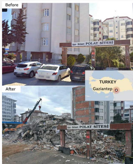
Edificio colapsado en Gaziantep Collapsed building in Gaziantep Fuente/Source: BBC Images
